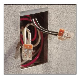
WALL-NUTS<sup>™</sup> are perfect for new construction and retrofit work.
