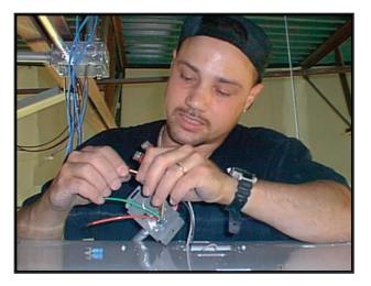
WALL-NUTS<sup>™</sup> work with solid and stranded wire making main, branch and fixture hookup fast, easy and safe.
