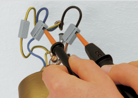
Testing through separate test slot
