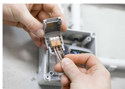
Place the wired connector in the Gelbox.
