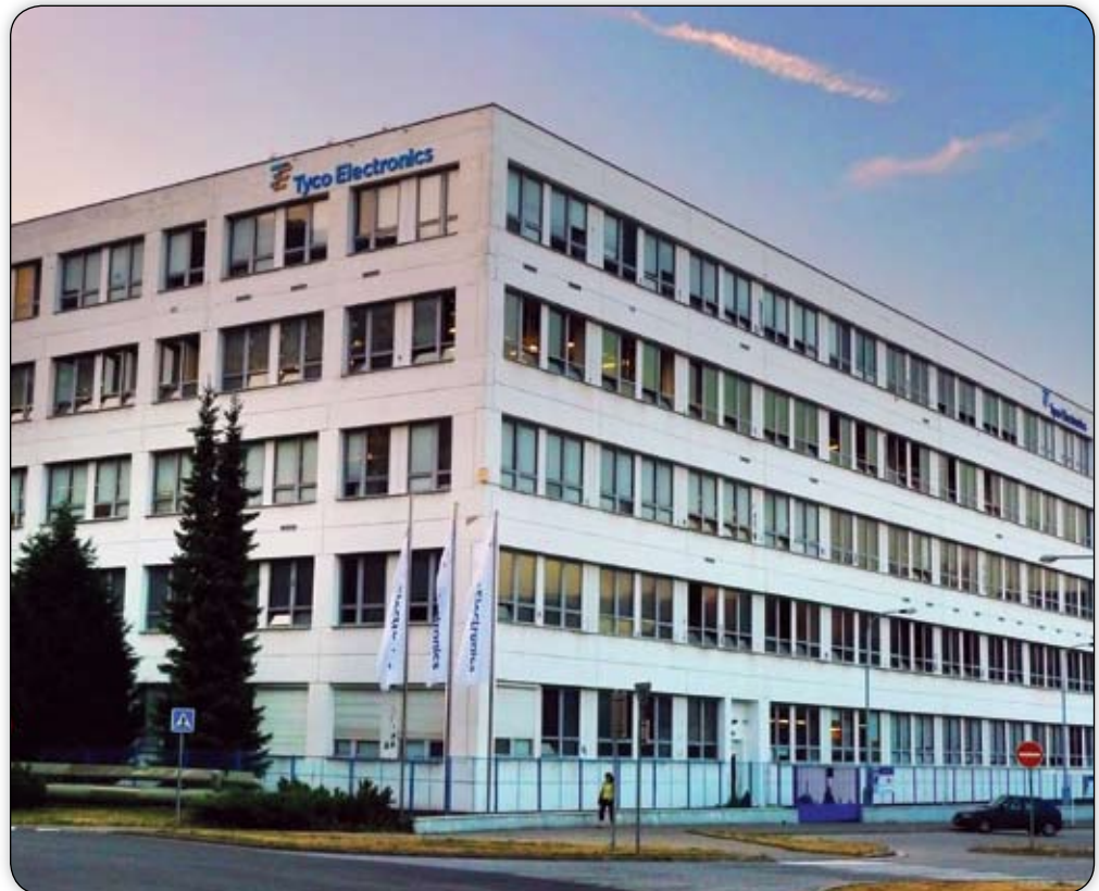
Tyco Electronics Manufacturing Facility in Trutnov, Czech Republic
